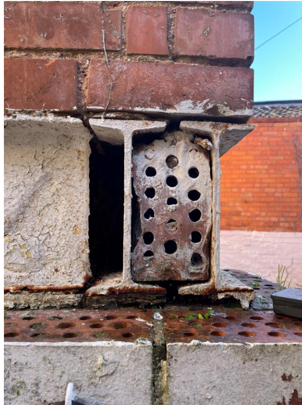
Figure 2: View of steels over SW column
